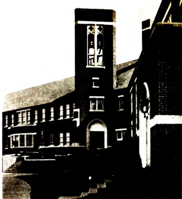
Nazarene Theological Seminary is in the process of building a $395,000 library, which would have been only thirty feet from the edge of the land the Junior College planned to condemn.
