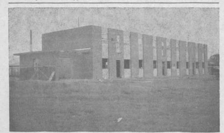
Construction is nearing completion on the newest men's dormitory, H. H. Wise Hall. The two story building will house forty-eight men. Of brick and concrete block construction, the dormitory will consist of six suites, three on each level. Each suite contains four two-man bedrooms, a lobby area, and bath. Only upper classmen will be permitted to reside in the dormitory.
