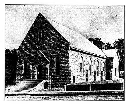
We are presenting herewith a picture of the new stone church which our people at Monterey, Tenn, have just completed. The erection of the building required more than a year's time. The stone for the building was quarried near, the work and the hauling being largely donated by members of the congregation. It is estimated that a duplicate of this building in Nashville, or in any city where everything had to be paid for, would cost around \$75,000.
