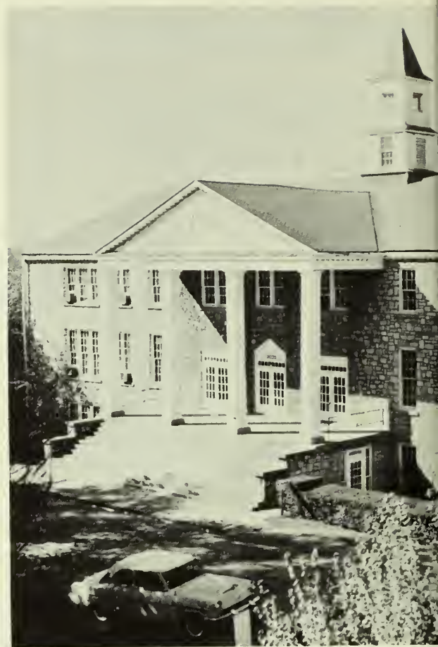
McClurkan Memorial Building
