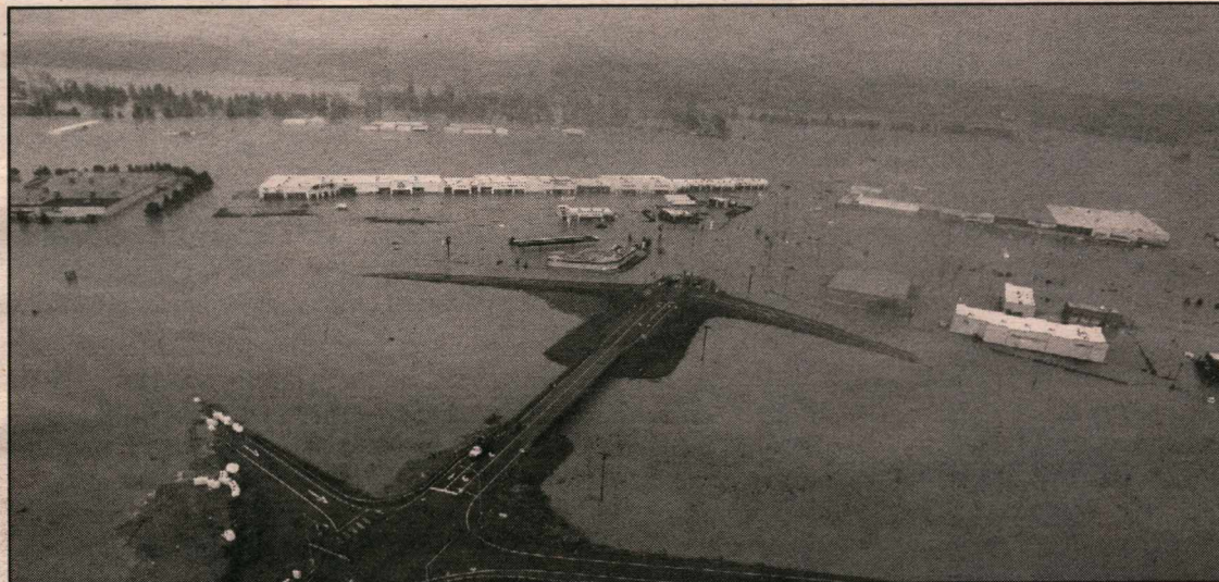
This is the overpass in Chehalis at exit 77 looking west over a shopping center completely under water including Wal Mart on the right. Interstate 5 goes below the overpass--it's completely submerged Tuesday, Dec. 4, 2007, in Chehalis, Wash. (photo by Associated Press).
